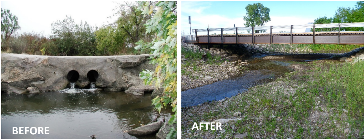
Replacement of perched culverts with a span bridge on Clear Fork Creek, Pottawatomie County
